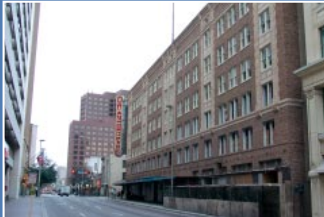
San Antonio EZ facility bonds are helping to renovate the 80 year-old Aztec Theater in the heart of downtown. (page 55)
