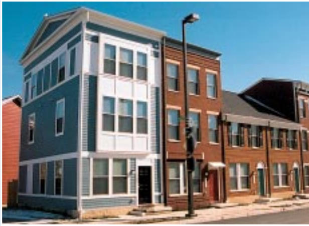
Albemarle Square features 340 units for rent and ownership. The Baltimore EZ helped to facilitate the resident engagement effort and land use plans.
