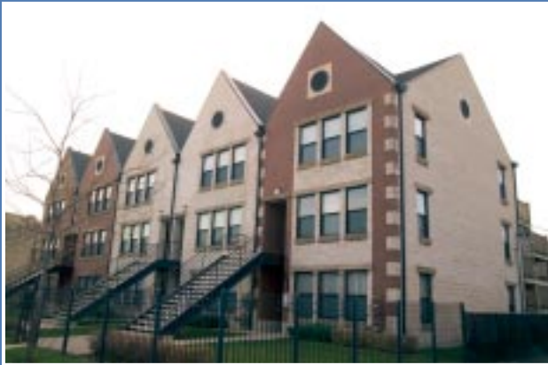
The Hearts United Housing EZ Social Services Block Grant funds are used to leverage additional funds and construct new housing units.
