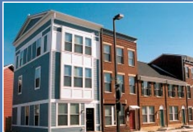
Albemarle Square has 340 units for rental and ownership. The Baltimore EZ helped to facilitate the resident engagement effort and land use plans.
