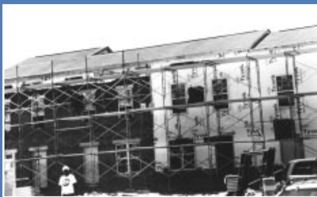
New housing being constructed in the Empowerment Zone.
