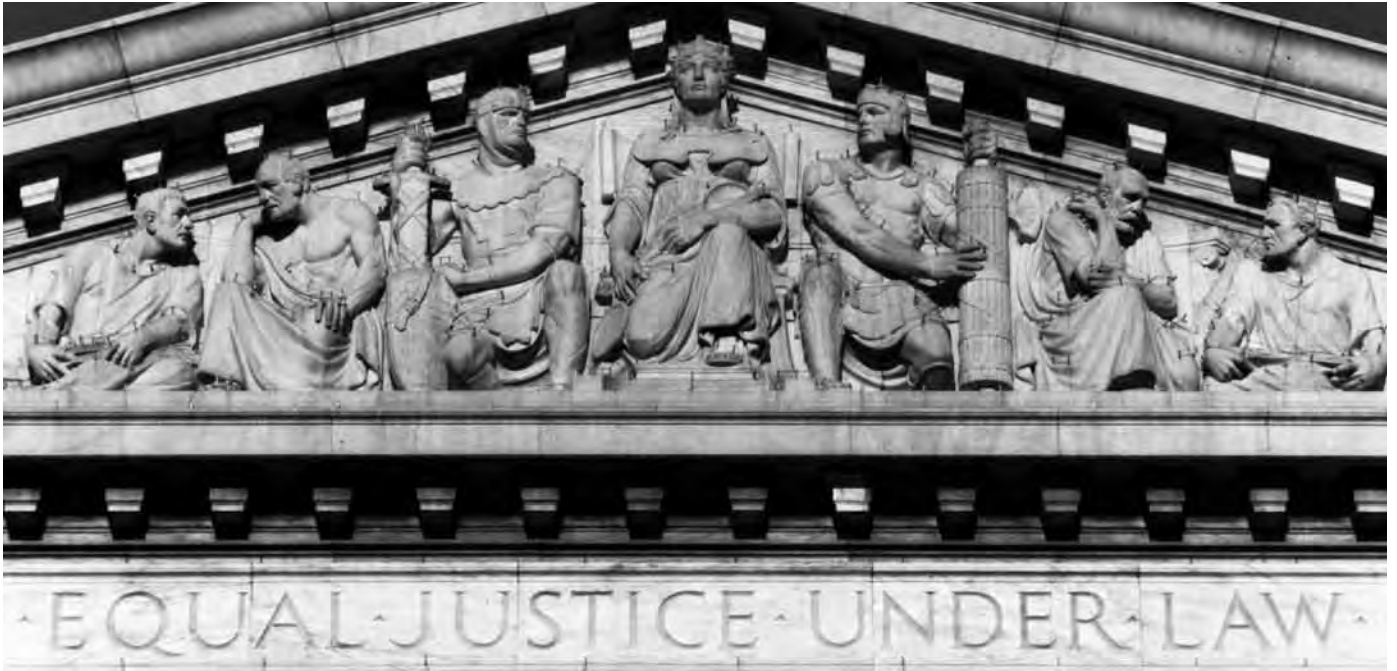
West Pediment Detail, Supreme Court Building. Photograph by John Neubauer. Courtesy of the Collection of the Supreme Court of the United States.
