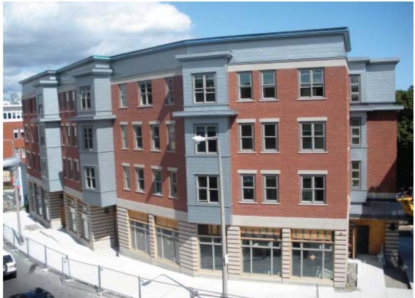
The Dudley Village project developed by the Dorchester Bay Economic Development Corporation in Boston will bring 50 affordable housing units to Roxbury.
