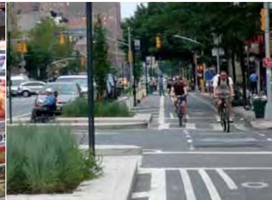
The protected bike lane on 9th Avenue was installed in fall 2007. In its first year, crashes involving all street users were down 56 percent, while bicycle ridership along the avenue increased 50 percent.
