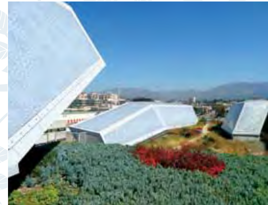
The Art Center College of Design's South Campus building, originally a 1940s-era aircraft testing facility, has been renovated as a LEED-certified green building featuring a roof-top garden with drought-resistant plants to reduce stormwater runoff.
