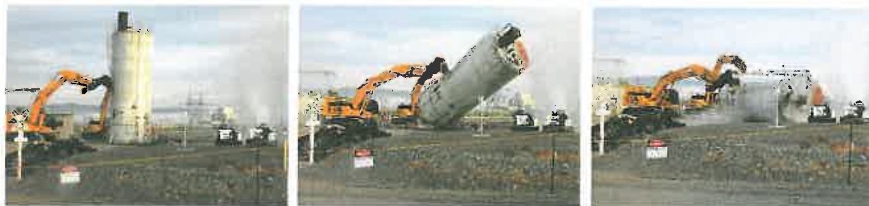
100 K Area Water Silo Demolition
