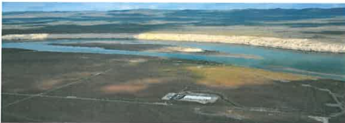
100 Area Groundwater Treatment Facility
