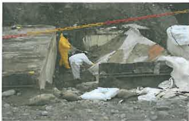
Removal of Waste Container from Burial Ground
