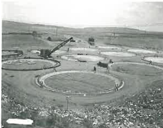
Construction of Hanford Tank Farm
