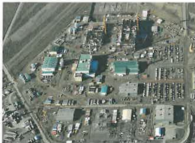
Waste Treatment and Immobilization Plant (Spring 2011)
