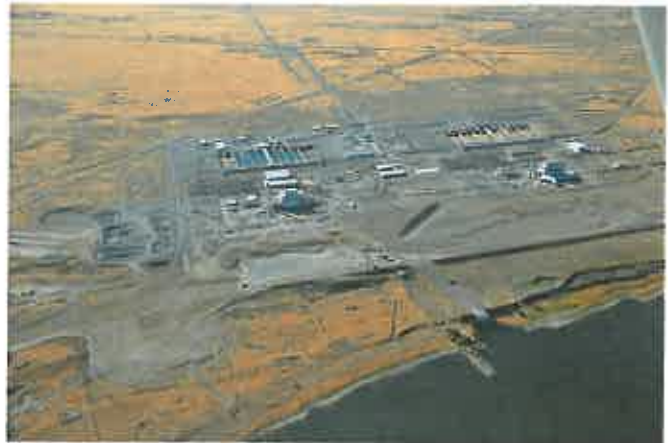
K East and K West Reactors
