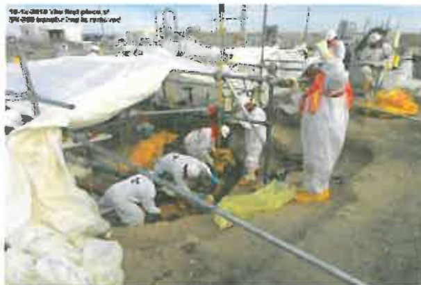
Transfer line being removed
