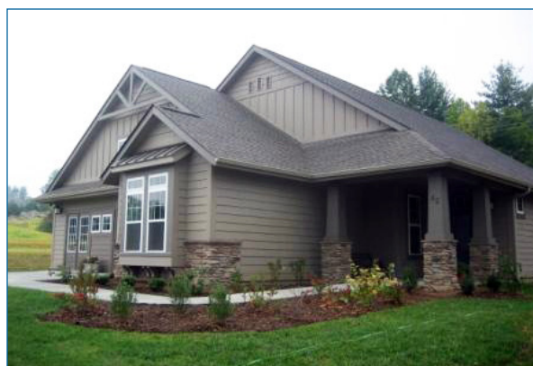
Nappier & Turner Co., Inc. completed the second WaterSense labeled new home during the pilot in early 2009.
