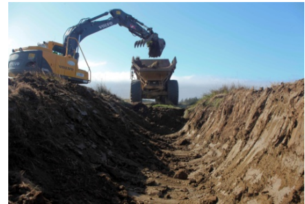
Channel digging (Roy Lowe/FWS).
