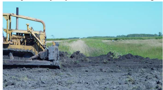
A bulldozer fills a drainage ditch as part of a wetland restoration on the Glacial Ridge property (TNC).
