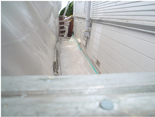
FIGURE 8.14 Exterior containment of polyethylene sheeting lines the narrow walkway between two houses. Notice the abatement worker in the background.
