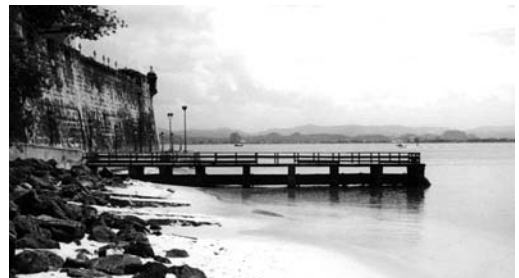
Point sources deliver pollutants to estuaries through a pipe or other discharge point. Here, the pipe is located under a pier (photo by R. Ohrel).
