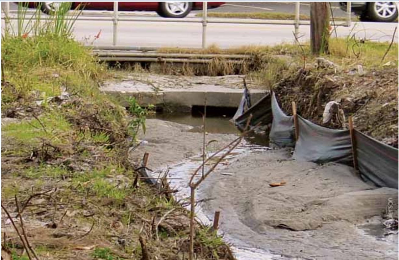
Urban stormwater runoff deposits large amounts of sediments and other pollutants into Sarasota Bay through drainage ditches (above) and tributaries (Gary Raulerson, SBEP).
