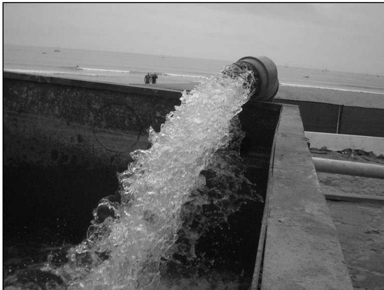
Photograph 11. Discharging from SL-1 during pumping (March 26, 2006).
