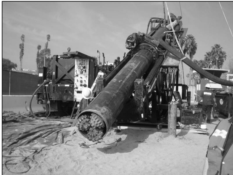
Photograph 2. Preparation to begin drilling of a 24-inch borehole (February 4, 2005).
