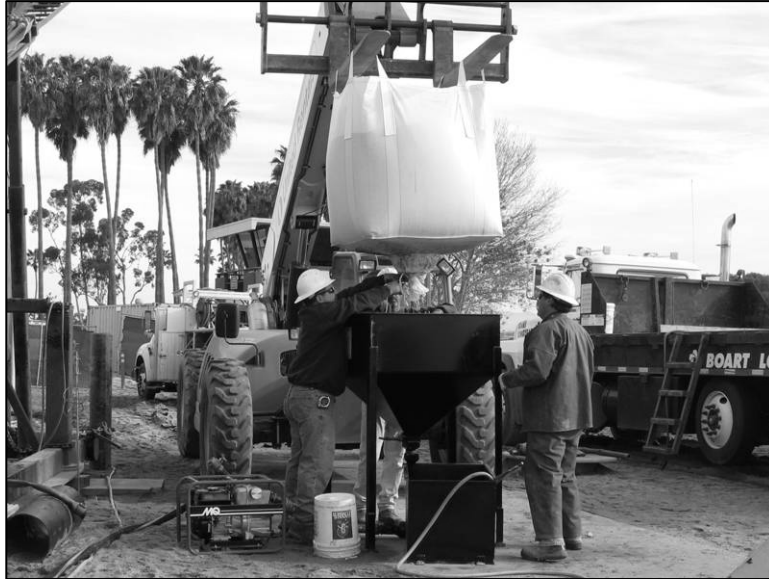
Photograph 7. Installing filter pack (March 5, 2006).
