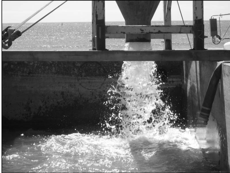
Photograph 9. Discharging during initial development by airlifting and swabbing (March 15, 2006).
