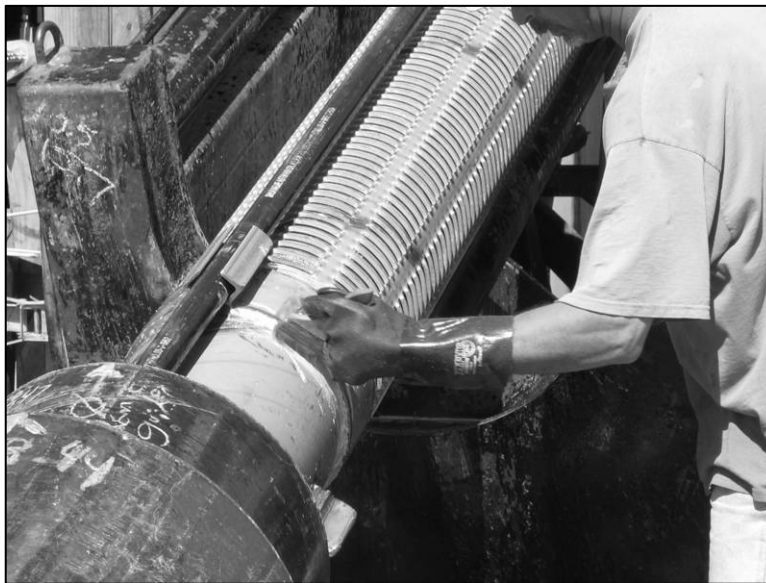
Photograph 6. Passivating field welds (March 1, 2006). Note tremie pipe at 12:00 position.
