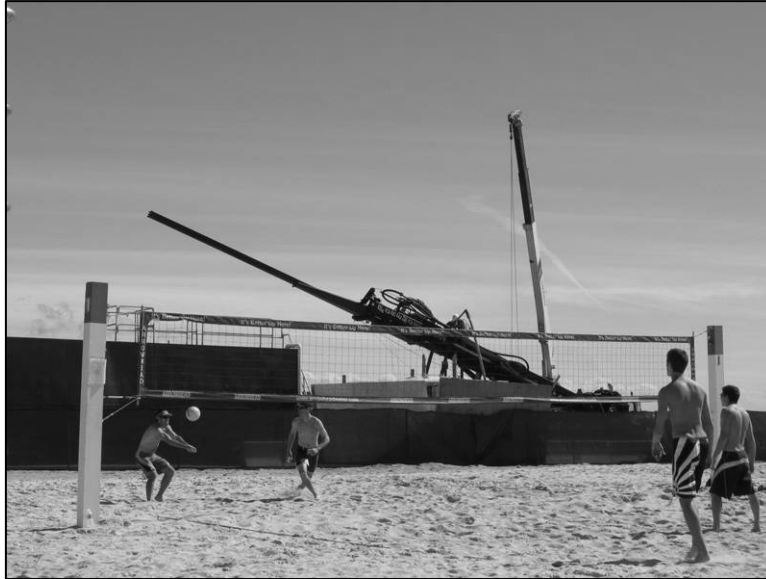
Photograph 1. Drilling rig set up on the beach (February 18, 2006).
