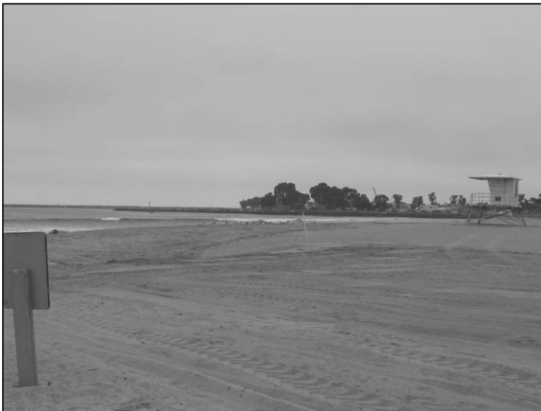
Photograph 15. Beach drilling site following demobilization.
