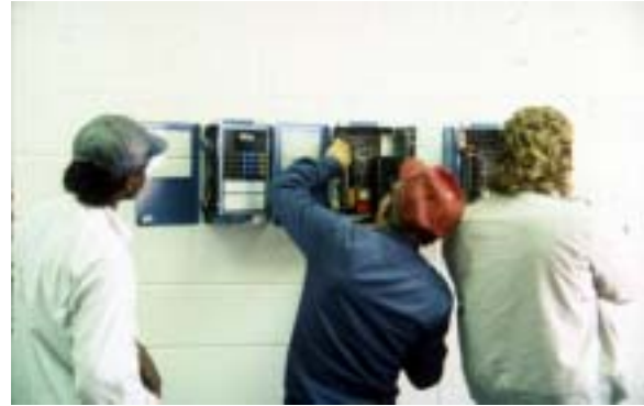
Control strategies, like CO sensors, help reduce energy loads by preventing equipment from operating when not necessary. NREL/PIX 11332
