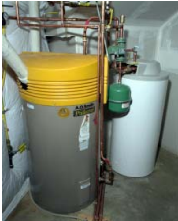
This central, high-efficiency boiler supplies hot water to two insulated storage tanks, providing hot water to six baths and a radiant floor heating system. NREL/PIX07925
