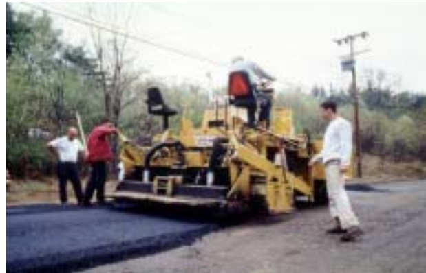
Concrete manufactured with flyash can be used for paving. NREL/PIX04358
