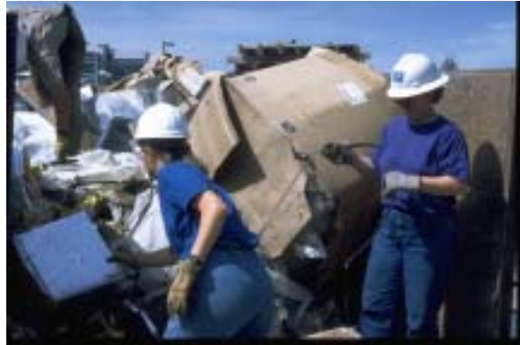
A construction site waste audit can help reduce waste generated and divert materials through processes from disposal through reuse and recycling. NREL/PIX 11407
