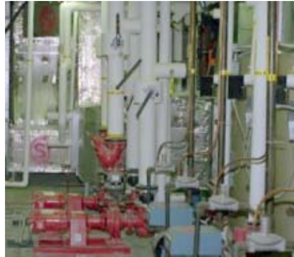
These loop water pumps and piping are part of a geothermal heat pump system being used by Nebraska schools to save money and energy on heating and cooling. NREL/PIX07415
