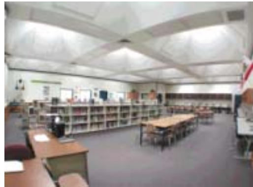
Deeply coffered ceiling helps to diffuse light from four skylights. There are no electric lights on in this photo. NREL/PIX 11470
