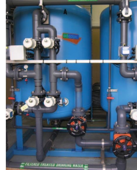
Small-scale arsenic removal technology filter system, part of EPA's Arsenic Demonstration Program
