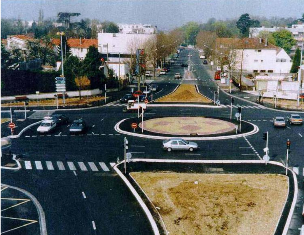
Figure 5. Signalized roundabout in France where crosswalks are located adjacent to the circular roadway. Note that France only allows post mounted signals. It is possible that overhead signals may be used in the US.(19)
