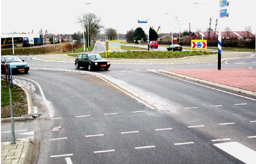
Figure 9. Typical juxtaposed pedestrian and bicycle crossing at a turbo-roundabout (22).
