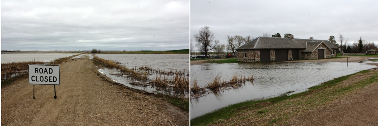
Flooding at Long Lake NWR forced closure of roads and other facilities in 2011.
