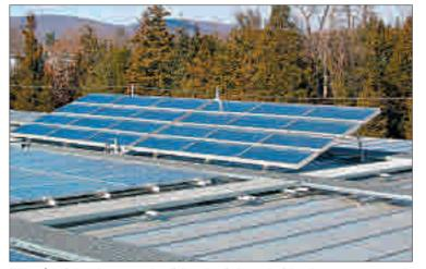
Water for sinks, showers and a dishwasher is heated with solar energy captured by solar panels on the building's roof.
