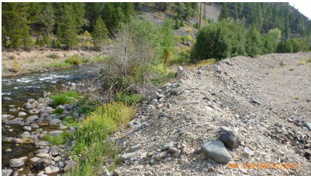
Photograph No. 7. View to the south looking downstream at a levee along river right that has been push-up to protect a gravel processing plant from floods. Yankee Fork of the Salmon River, Yankee Fork Subbasin, Idaho – Bureau of Reclamation Photograph by P. Drury, September 12, 2011.
