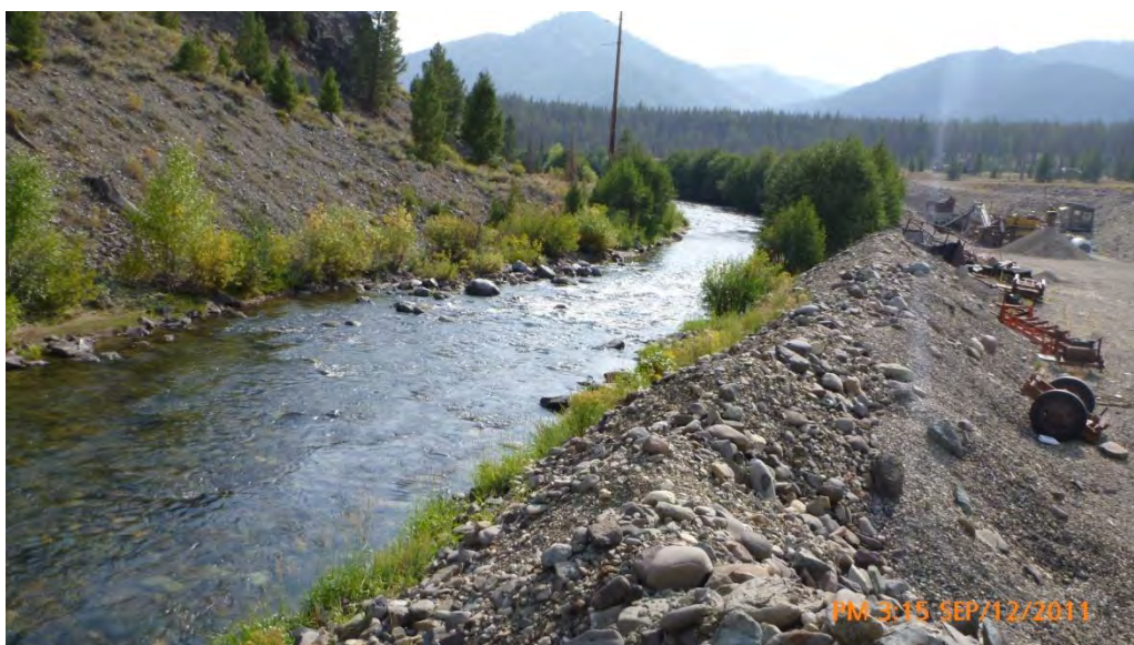
Photograph No. 12. View to the southwest looking downstream along a levee that has been pushed-up to protect a gravel processing operation along river right. Yankee Fork of the Salmon River, Yankee Fork Subbasin, Idaho – Bureau of Reclamation Photograph by P. Drury, September 12, 2011.
