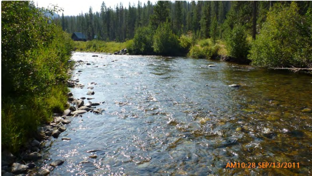
Photograph No. 49. View to the southeast looking downstream at a rock revetment (left of center) that was placed at the head of a side channel. An overflow channel has developed just left of the revetment. West Fork of the Yankee Fork of the Salmon River, Yankee Fork Subbasin, Idaho – Bureau of Reclamation Photograph by P. Drury, September 13, 2011.
