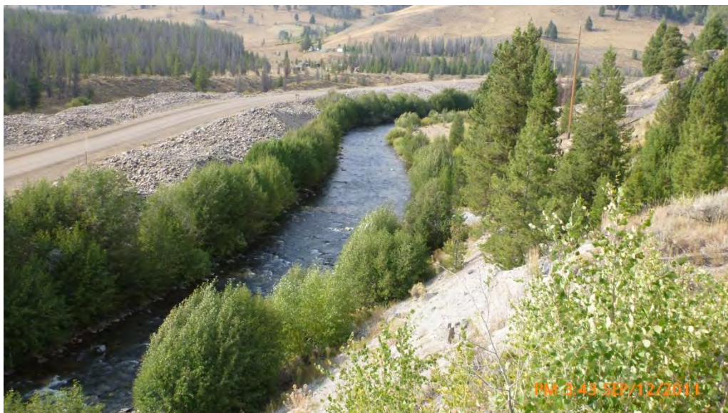
Photograph No. 15. View to the north looking upstream at a plane-bed channel that is confined between dredge tailings (river right) and colluvial deposits (river left). Yankee Fork of the Salmon River, Yankee Fork Subbasin, Idaho – Bureau of Reclamation Photograph by P. Drury, September 12, 2011.
