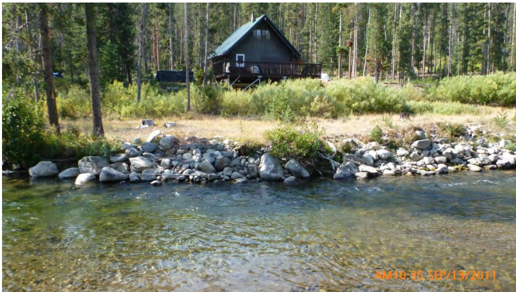
Photograph No. 53. View to southwest looking across the channel at bank armoring placed along river right and lateral scour pool. West Fork of the Yankee Fork of the Salmon River, Yankee Fork Subbasin, Idaho – Bureau of Reclamation Photograph by P. Drury, September 13, 2011.
