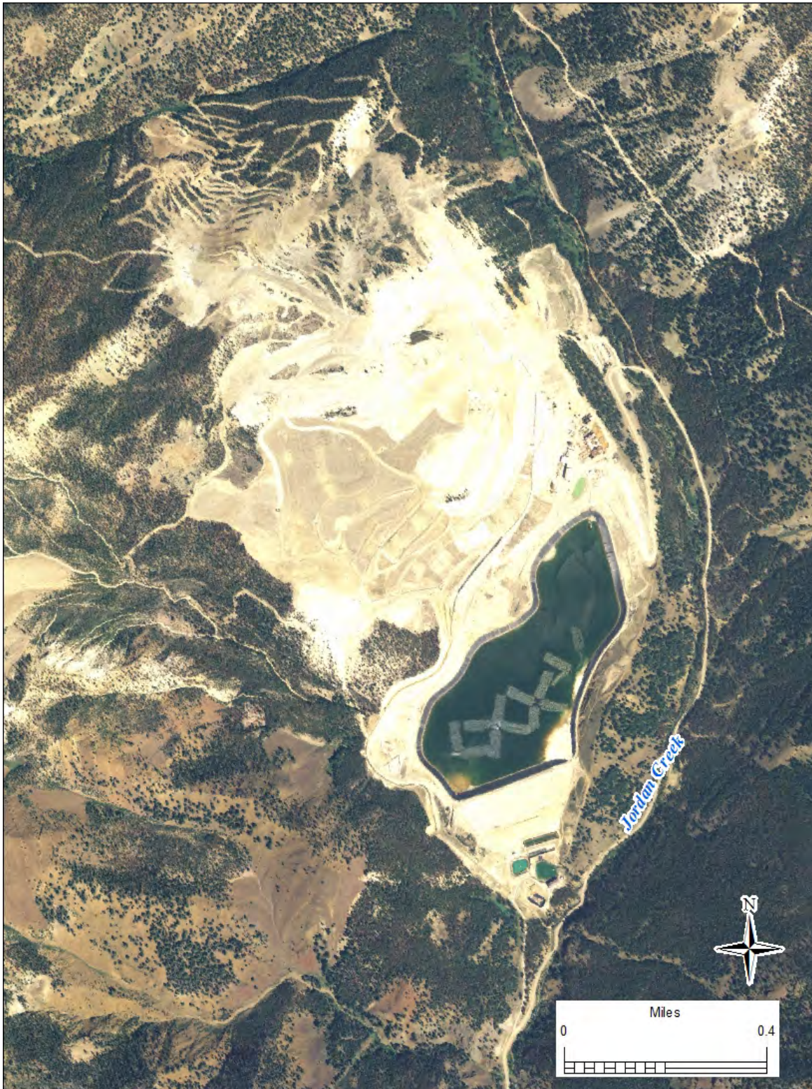
Figure 9. Grouse Creek Mine that was operated by Hecla Mining along Jordan Creek in 2009.
