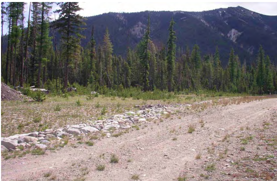
Figure 6-8. The staging and stockpile area for the Bumping Lake adult collection facility is in an already disturbed area below the dam.
