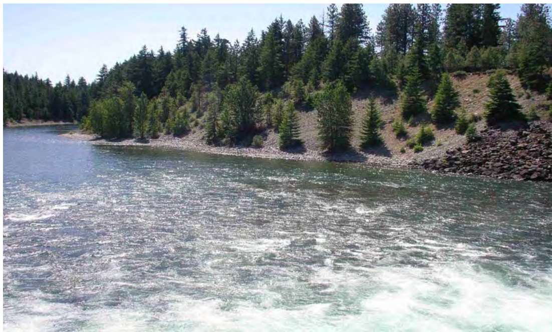
Figure 6-3. Immediately downstream of Cle Elum Lake Dam - the vicinity where the barrier dam would be constructed.
