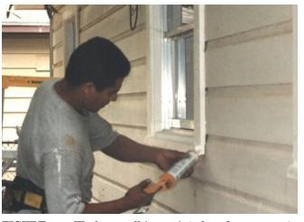
FIGURE 3.3 Worker caulking painted surfaces as part of ongoing lead-safe maintenance.
