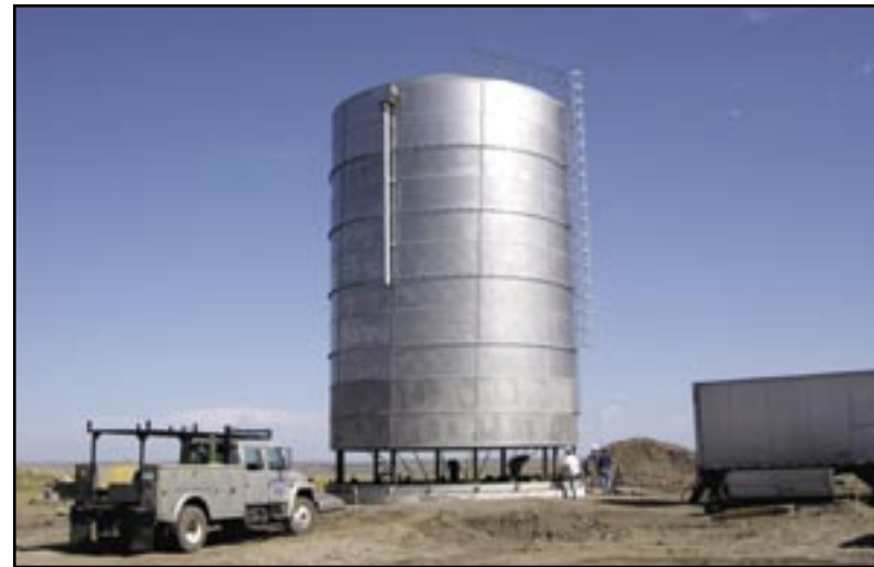
Figure 10: New 300,000-gallon stainless steel reservoir.
