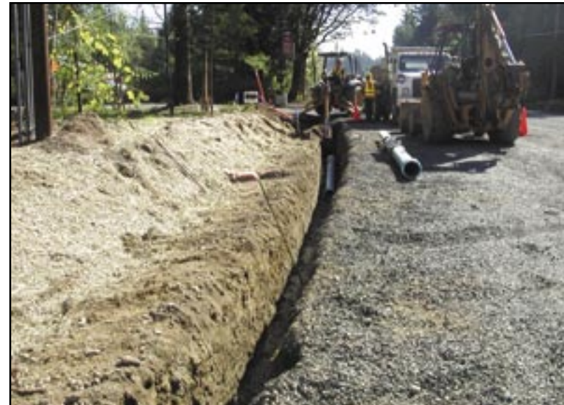
Figure 29: 8" PVC water main installation.
