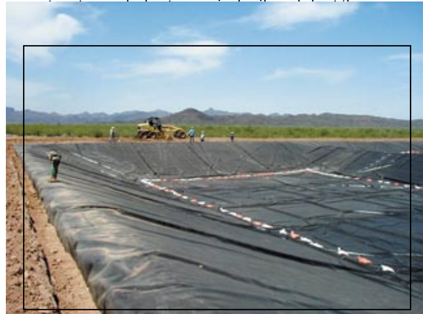
Figure 19: Anchor trench installation.
