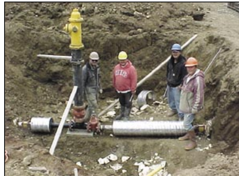
Figure 36: Waterline repair project in Toksook, Alaska.
