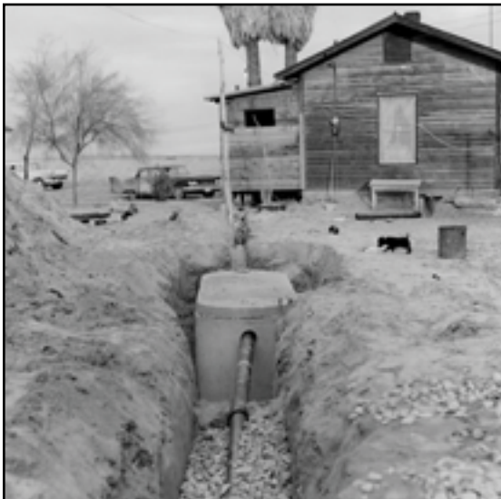
Figure 1: Construction of a septic system, 1960's.
