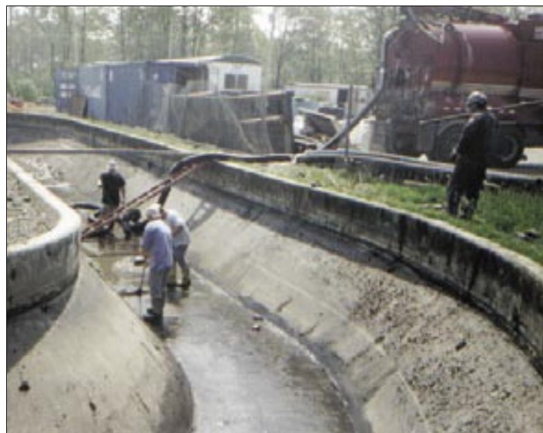
Figure 8: Cleaning an oxidation ditch in Penobscot, Maine.
