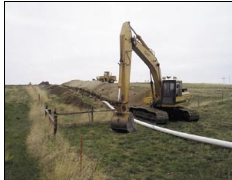
Figure 11: Waterline installation.
