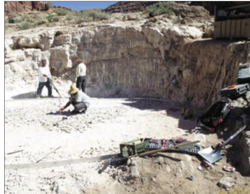
Figure 17: Construction of a new tank foundation.
