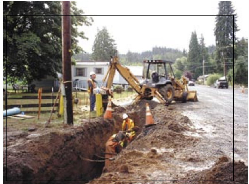
Figure 28: 8" PVC water main installation.
