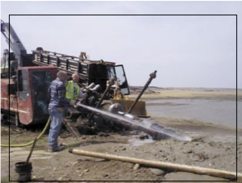
Figure 9: Directional drilling under the Grand River Arm of Lake Oahe.
