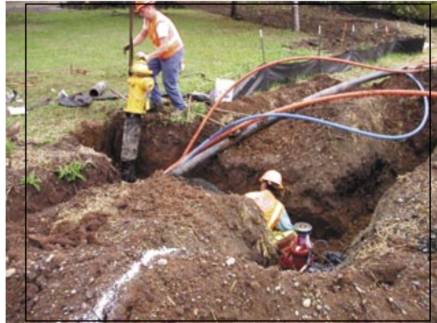
Figure 26: Hydrant installation.
