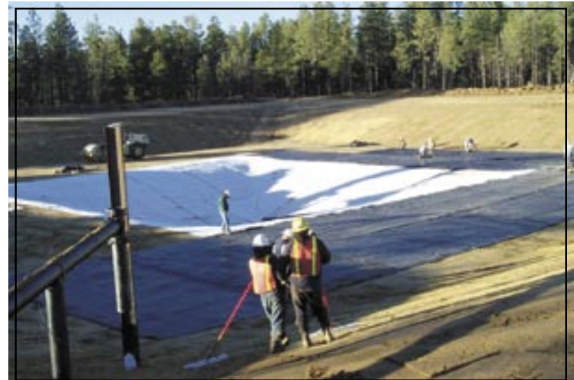
Figure 12: Installation of geosynthetic clay liner in a fermentation pond.
