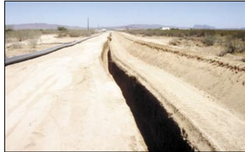
Figure 24: Sewerline trench.
