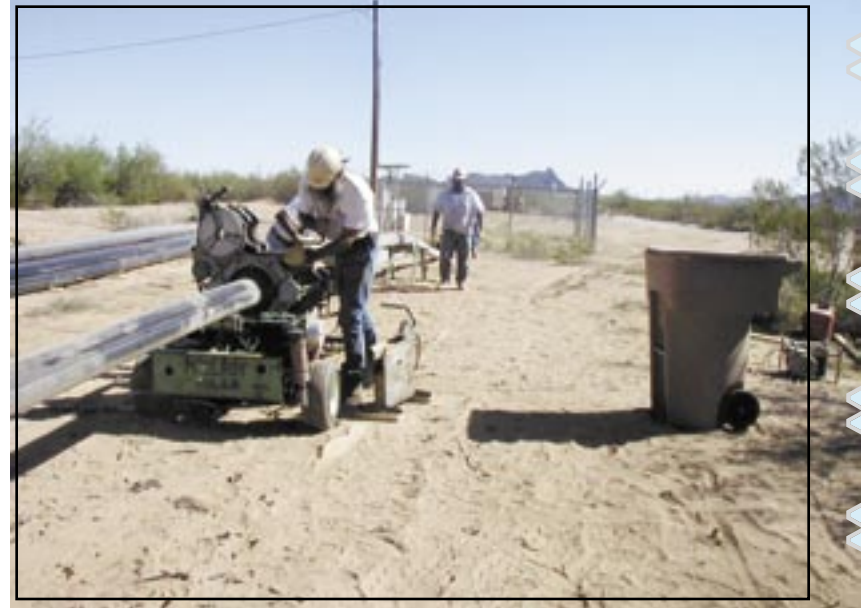
Figure 22: Fusing HDPE pipe.
