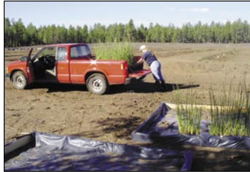
Figure 14: Installation of wetland plants.
