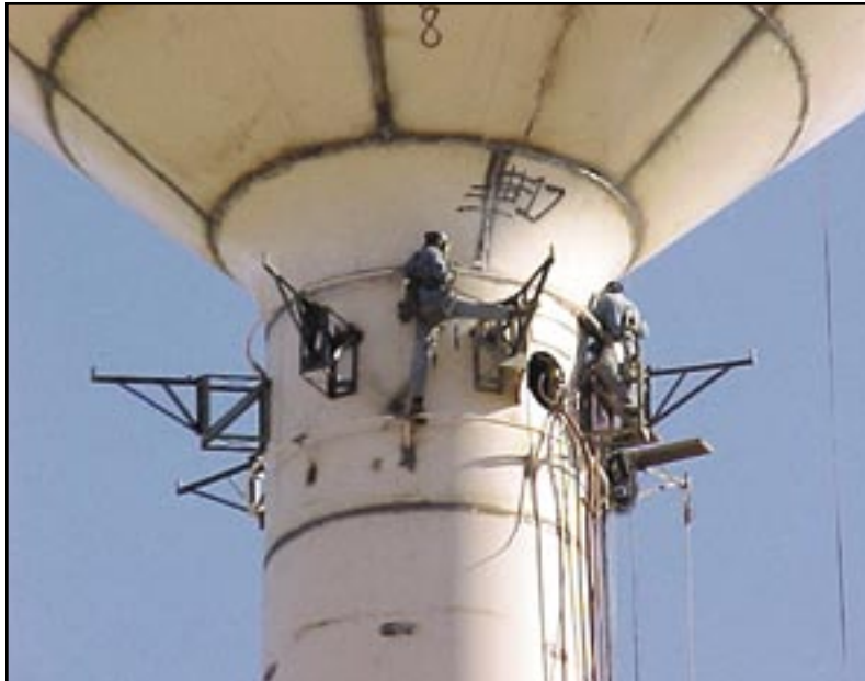
Figure 37: Welding on a watersphere in Cocopah, Arizona
