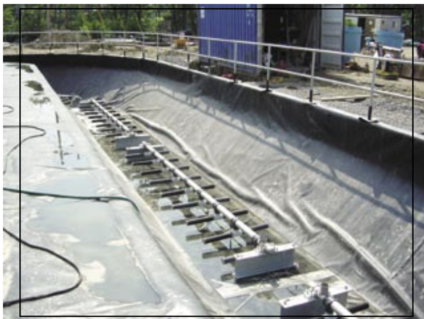
Figure 30: Wastewater treatment plant aerators construction in Penobscot Nation, Indian Island, Maine.
