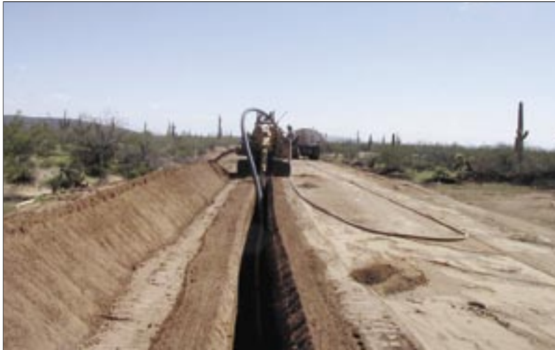
Figure 23: Laying HDPE pipe.
