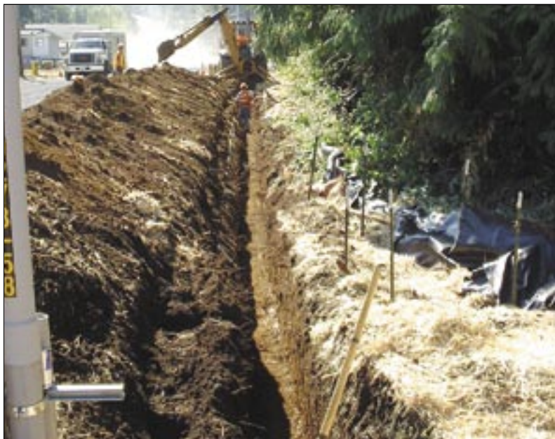
Figure 25: Water main trench.
