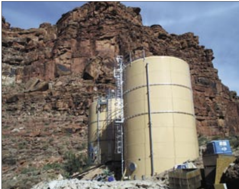
Figure 16: New 108,000-gallon water storage reservoir.
