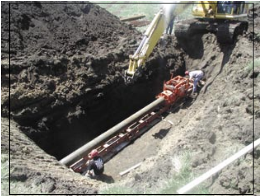
Figure 39: Road bore for a waterline extension, Winnebago, Nebraska.
