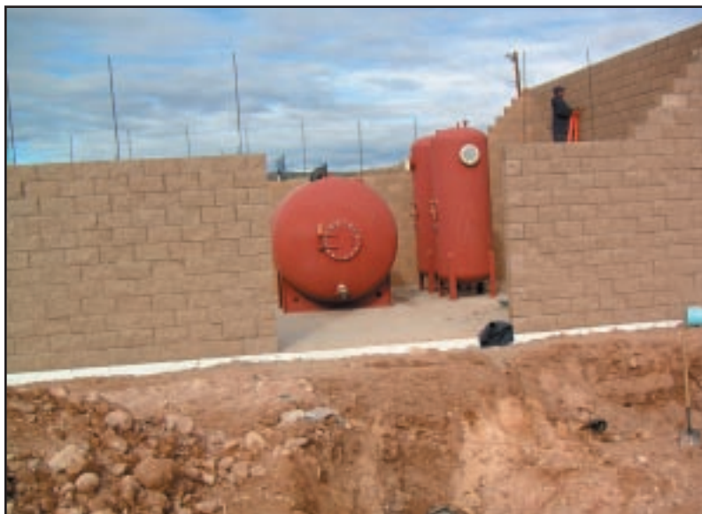
Figure 9: Jemez filtration installation during building construction.
