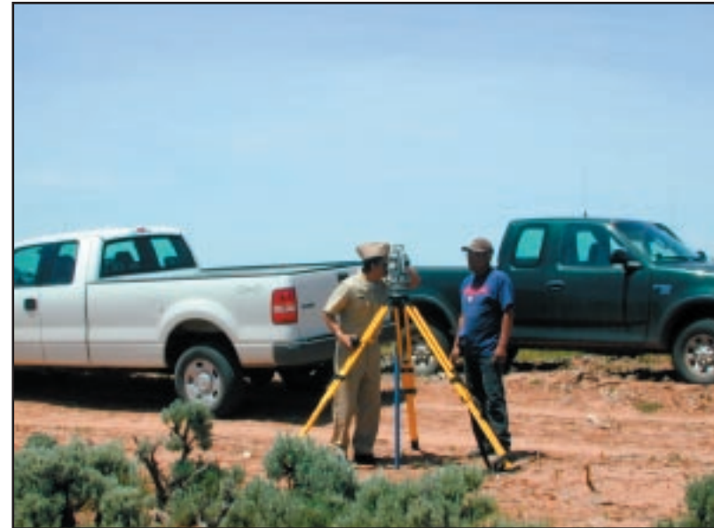
Figure 22: Surveying for the proposed extension.
