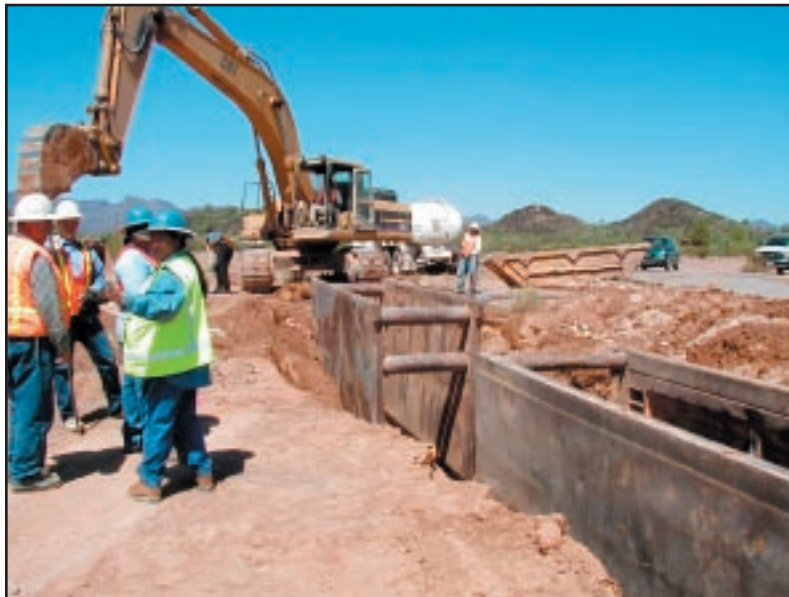
Figure 39: Trench box installation, Santa Rosa Village, Tohono O’odham Reservation.
