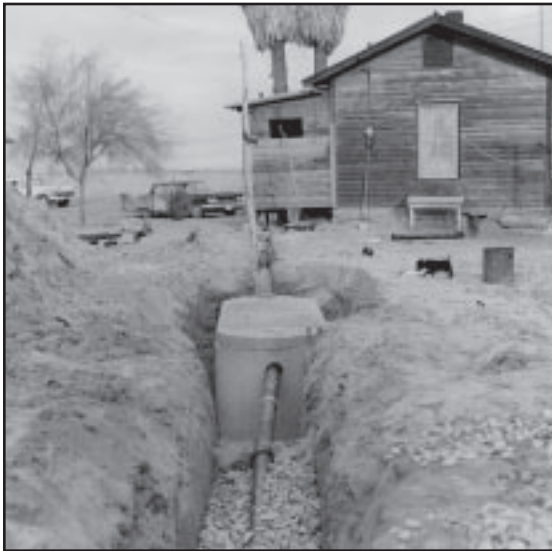
Figure 1: Construction of a septic system, 1960's.
