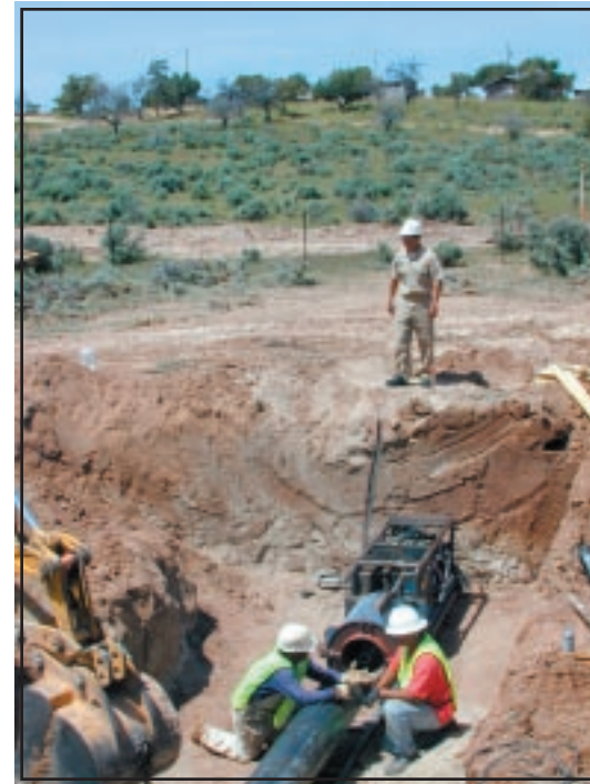
Figure 24: IHS Engineer inspects the road bore.
