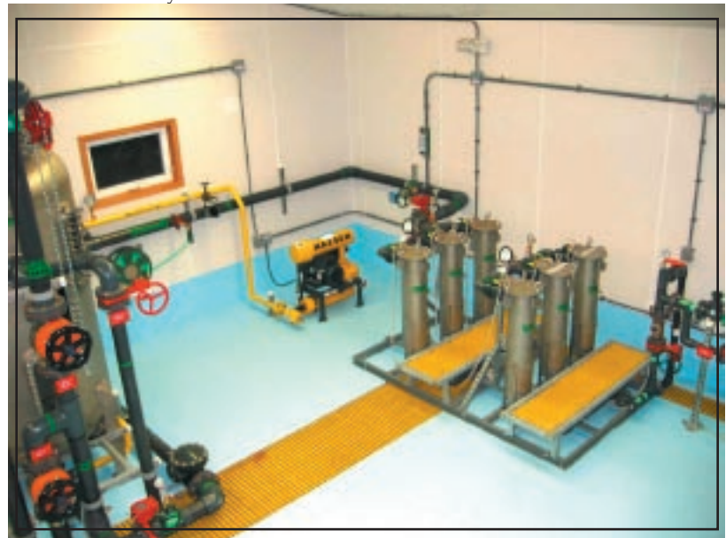
Figure 29: Tatitlek's new 1,200 sqft surface water treatment facility produces 36,000 gallons of potable water per day.
