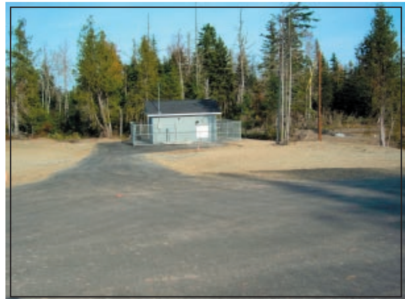
Figure 36: Completed lift station, Pleasant Point, Maine.
