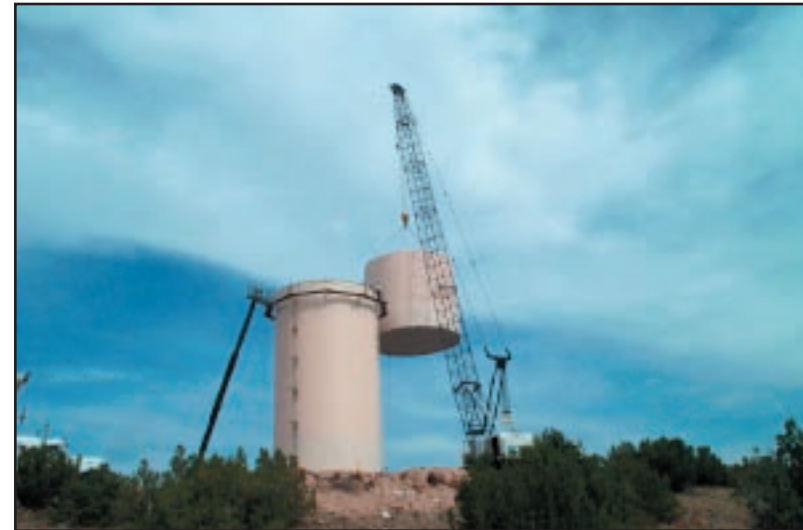
Figure 11: Jemez 365,000 gallon storage tank installation of the roof section.
