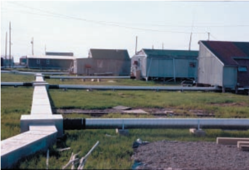
Figure 13: Permafrost (permanently frozen soil, commonly found in arctic regions) requires using aboveground water and sewer utilidors; service lines then branch off to connect to homes. 1
