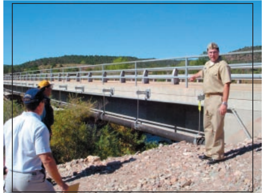
Figure 31: LT Chris Glime describes the design of a sanitary sewer bridge crossing to White Mountain Apache Utility personnel in Cibecue, Arizona.
