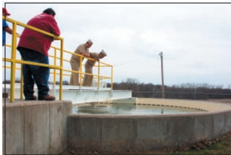
Figure 8: Sanitary survey at Kickapoo Tribe of Kansas water treatment plant performed by LT Joe Jones and LCDR David Hogner.
