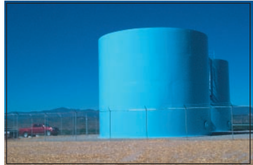
Figure 21: The two completed 250,000 gallon water tanks.
