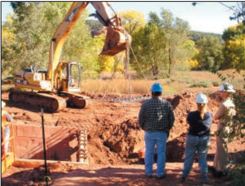
Figure 30: IHS engineers and inspector observe a lift station base reinforcement being placed under a lift station renovation project, Fort Apache Reservation.
