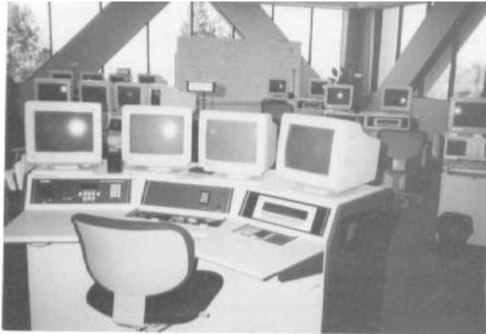
Exhibit 2-6. Los Angeles County's Command and Control Facility.
