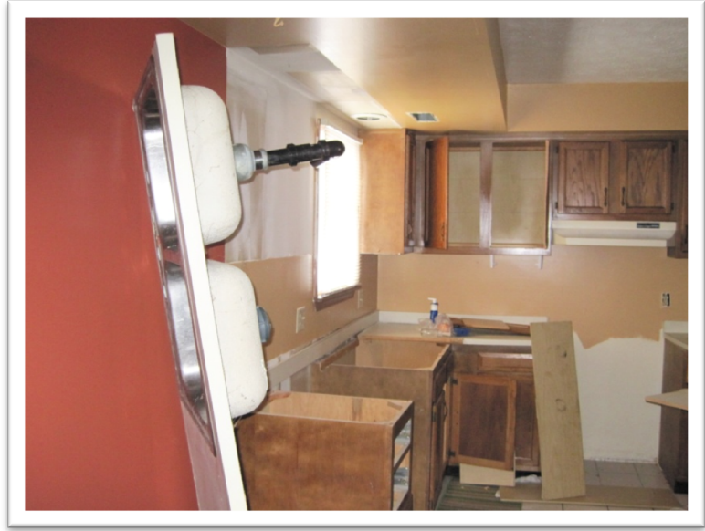
Figure 2: kitchen stripped of cabinets, with sink removed from counter
