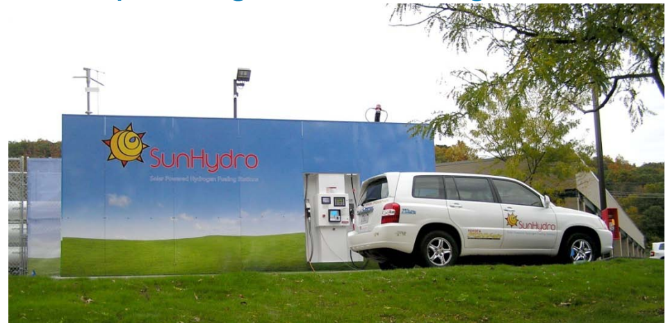
65 kg/day system, operating Proton fueling station
