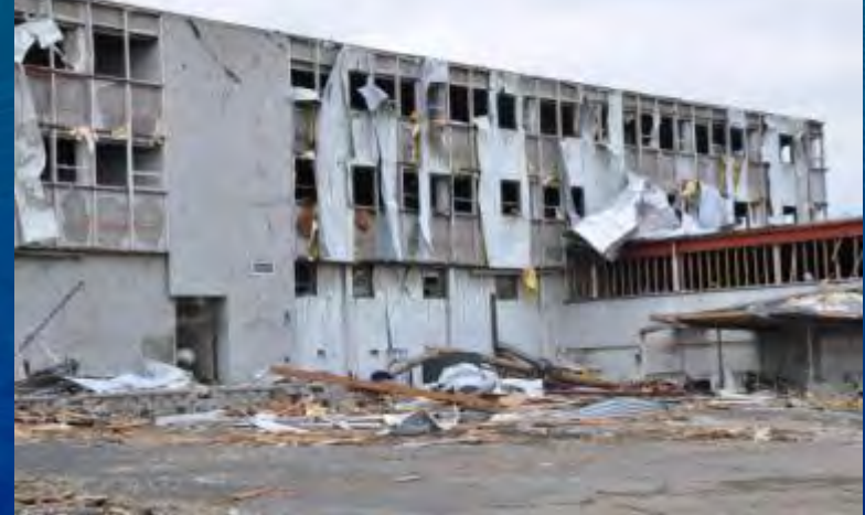
4-Story RC Frame Professional Building
