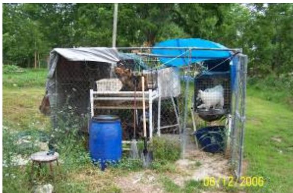
Shelter not structurally sound
