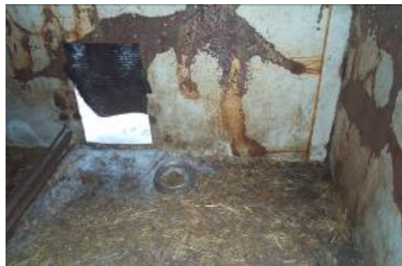
No bedding, rusted enclosure
