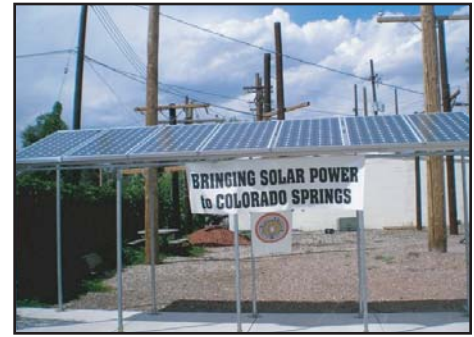
Finished solar panels installed by the apprentices of the Joint Apprenticeship Training Committee
