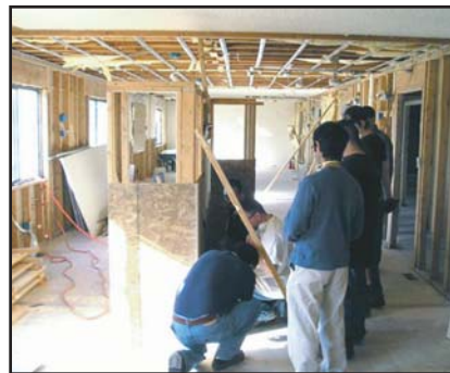
Green Crew learns framing at the Avalon worksite.
