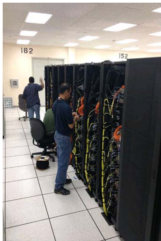
Gyre being installed in the Orlando, FL facility in early October 2012.
