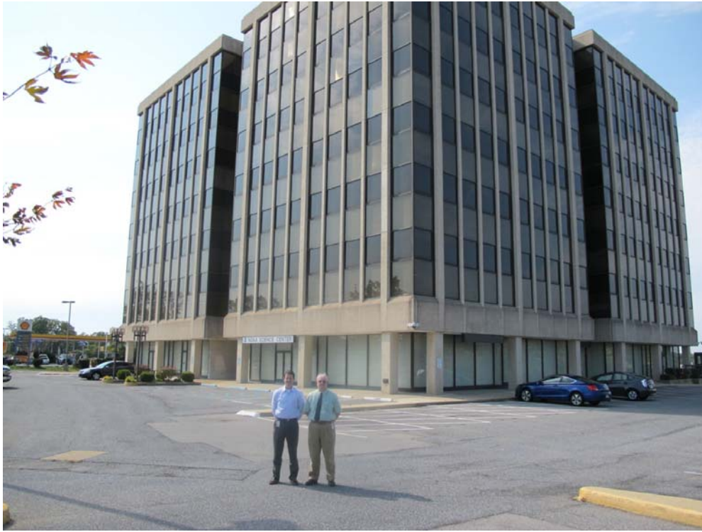
Wallace Hogsett (HPC Science and Operations Officer) and Ed Danaher in front of the WWB representing two extremes. Wallace worked at the WWB for a few days, and Ed for a few decades.
