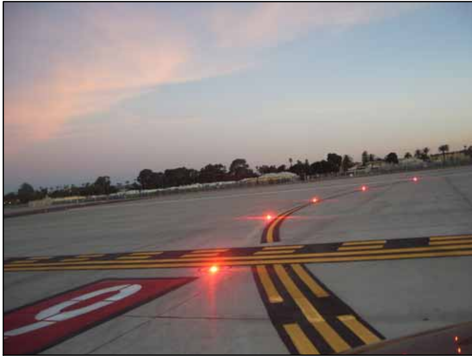
FIG 2-1-12 Runway Entrance Lights
