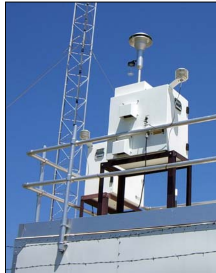
Air Monitoring Station
