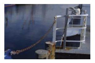
**Edges** of decks, platforms, flats, scaffolding, staging, runways, and similar flat surfaces that are more than 5 feet above a solid surface must be guarded with
