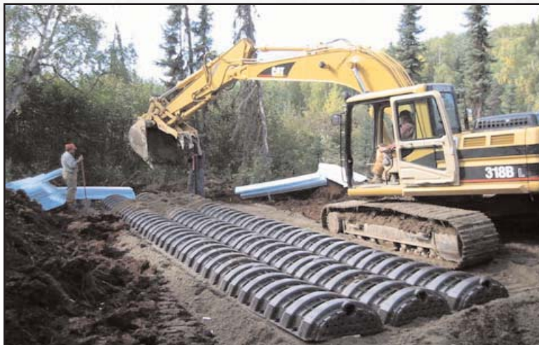
Figure 35: Sewer infiltrator sections installed in Alaska.
