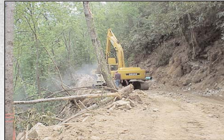
Figure 26: Mountainside installation, clearing the right-of-way.
