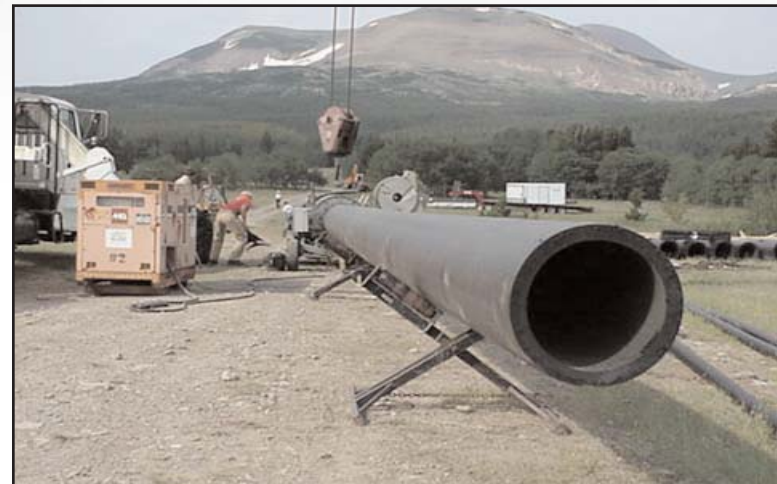
Figure 22: 22 inch line fuses together and 4 inch air valve fused together.
