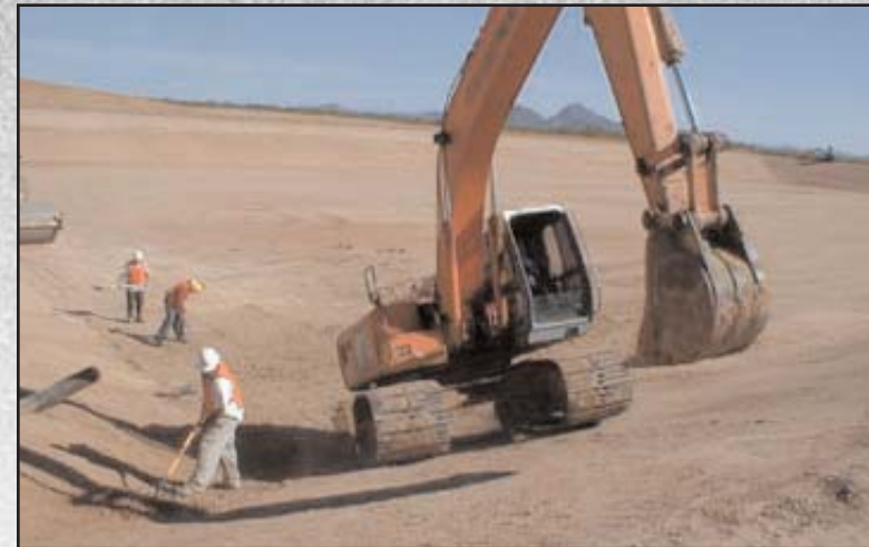
Figure 10: Preparing lagoon floor for liner expansion.
