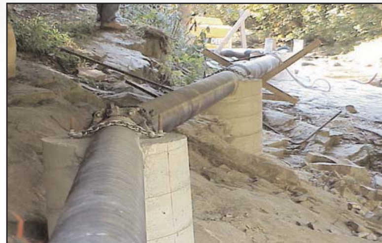
Figure 29: Pipe on piers under Straight Fork Bridge.
