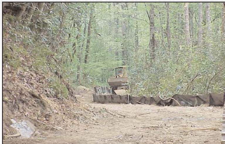
Figure 23: Cleared right of way with erosion control. Silt protection for nearby trout streams is essential.
