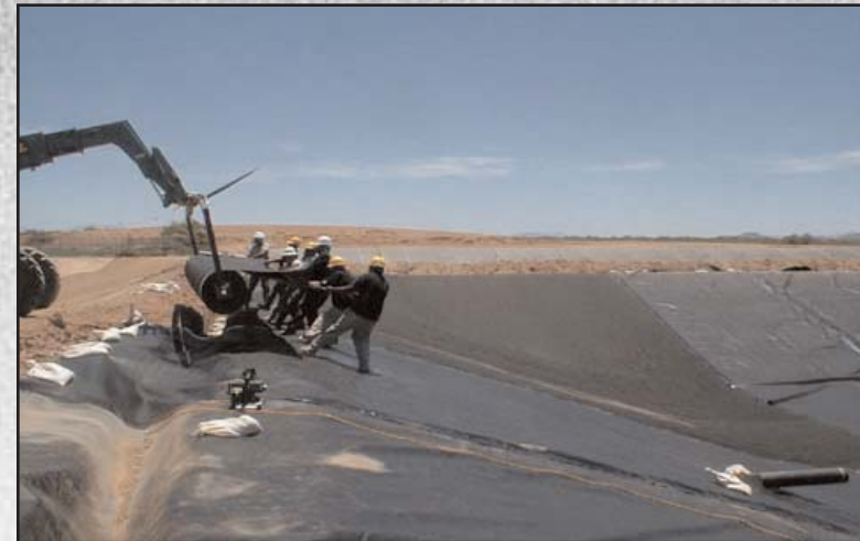
Figure 46: High density Polyethylene (HDPE) liner placement in expanded lagoon, Arizona.
