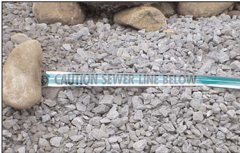
Figure 25: Sewer caution tape above Big Cover sewer line.
