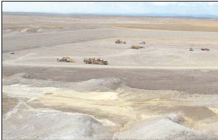
Figure 30: Construction of 10-acre landfill.
