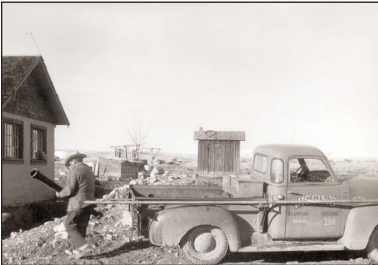
Figure 1: Construction of a septic system, 1960's
