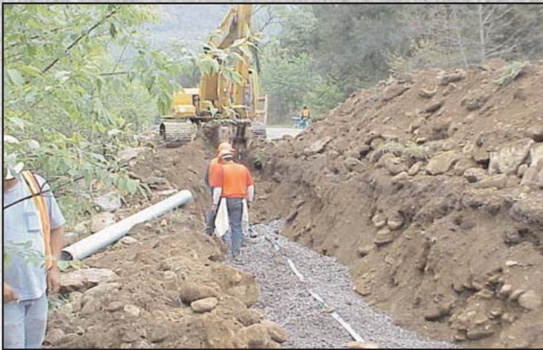
Figure 27: Big Cove Loop Road-8" PVC sewer lateral.
