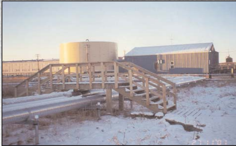
Figure 42: Vacuum sewer lines leading to a water treatment /vacuum sewer/washeteria building in Selawik, Alaska.
