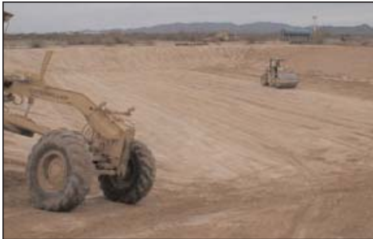
Figure 9: Construction of lagoon expansion cell.
