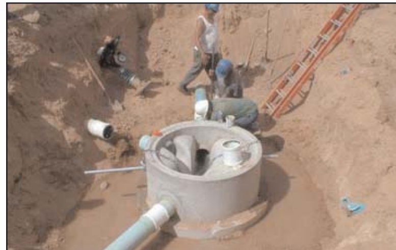
Figure 12: Sewer system expansion manhole construction.
