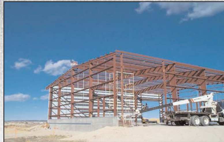
Figure 33: Steel siding going up on the Pine Ridge Baler Building.
