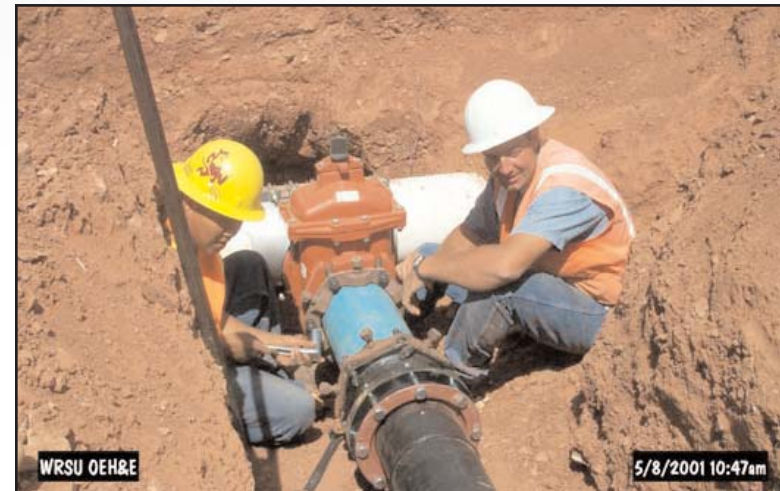
Figure 18: White Mountain Apache Tribal members made up majority of construction workers connecting the Cedar Creek system to the Whiteriver system.
