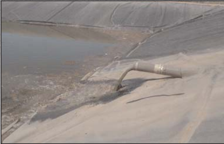
Figure 47: Wastewater flow into completed lagoon, Arizona.
