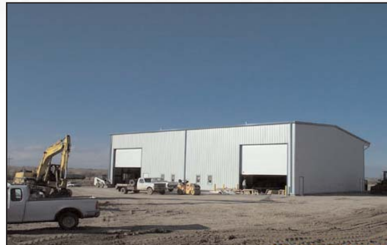
Figure 34: Completed Pine Ridge Baler Building
