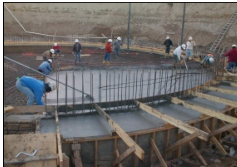
Figure 27: First quarter concrete pour for the clarifier base.
