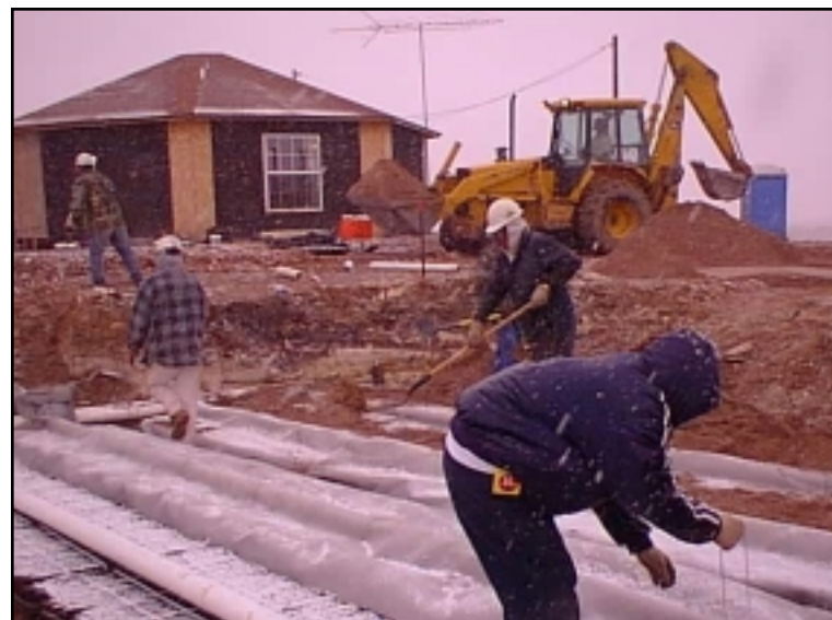
Figure 8: Septic tank and drainfield installation on the Navajo Reservation, Arizona.
