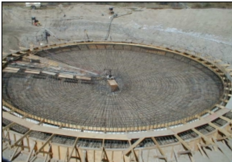
Figure 26: Rebar placement for the base of the clarifier.
