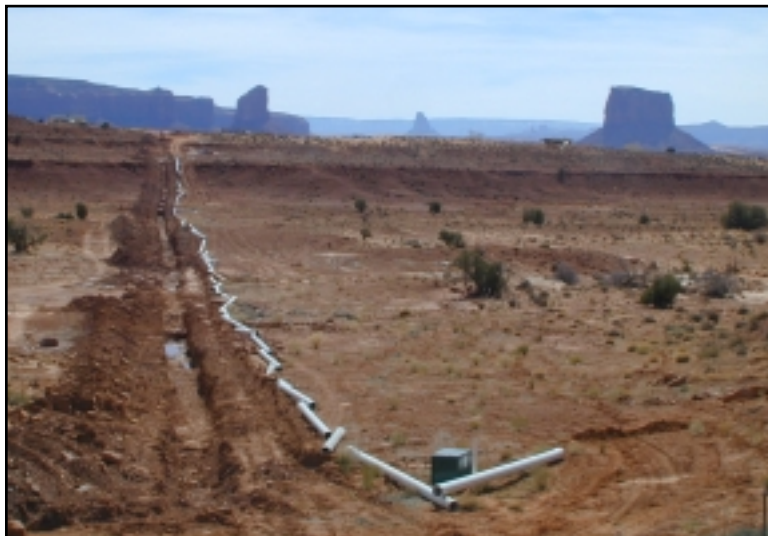
Figure 24: Waterline extension in Monument Valley, AZ.
