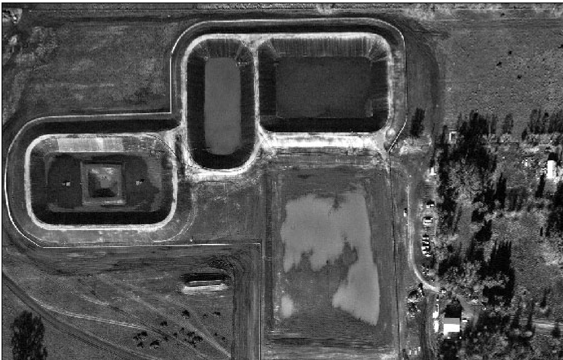
Figure 23: Aerial View of the AIWPS
