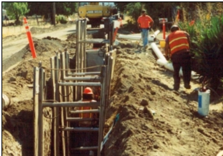
Figure 20: Sewer main construction on Tabor Road.
