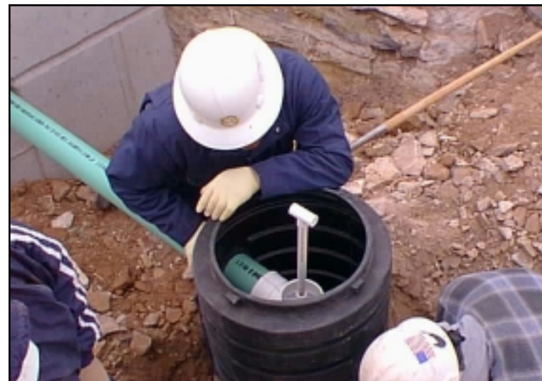
Figure 42: Drainfield control valve for multi-field system, Canyon de Chelly, AZ
