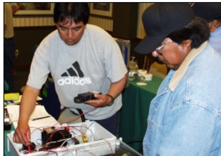
Figure 16: Team approach for solving electrical problems
