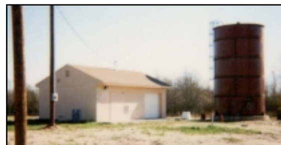
Figure 14: Completed pumphouse and clearwell tank
