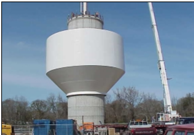
Figure 37: Construction of a water tank in Tunica Biloxi, MS
