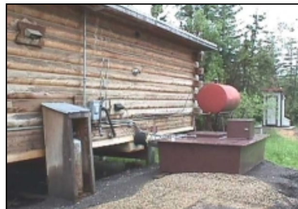
Figure 31: Flush and haul holding tank in Northway, Alaska.
