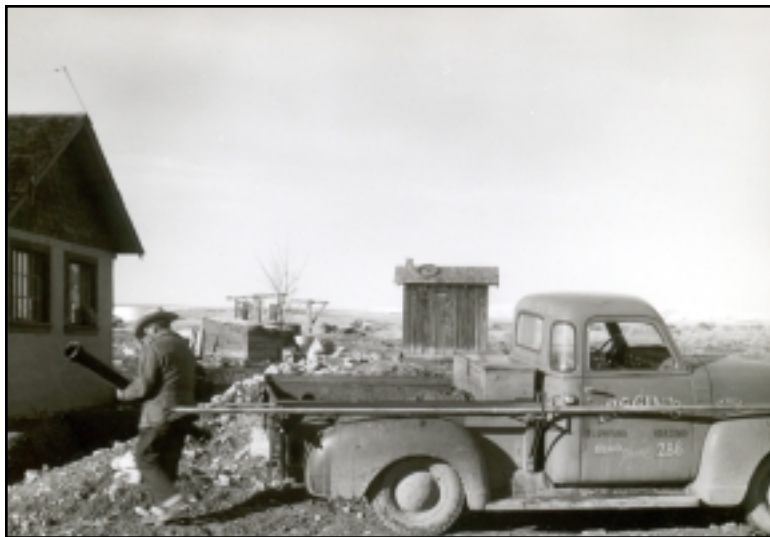
Figure 1: Construction of a septic system, 1960's
