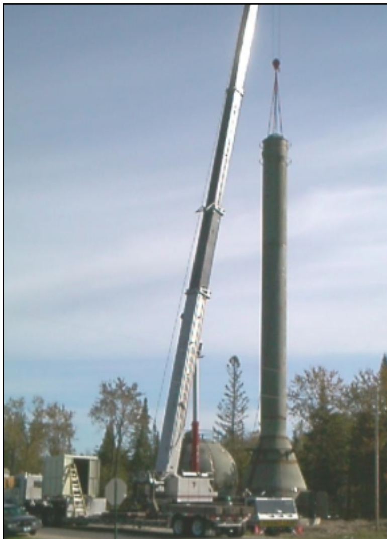
Figure 30: Erecting pedestal of 50,000 gallon elevated storage sphere, MN
