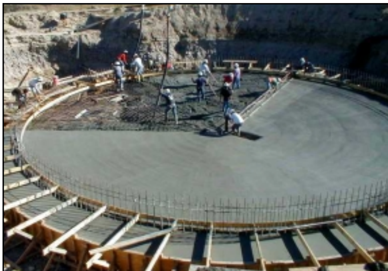
Figure 28: Concrete pour for the base of the clarifier.
