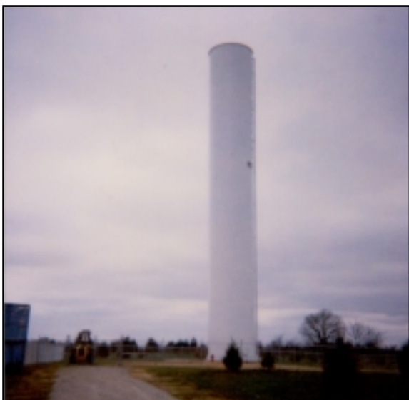
Figure 13: Completed 16' x110', 60,000 gallon stand pipe.
