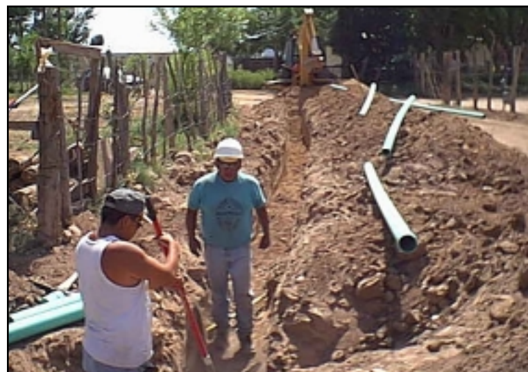
Figure 38: IHS contractor installing water service line, Santo Domingo Pueblo, NM
