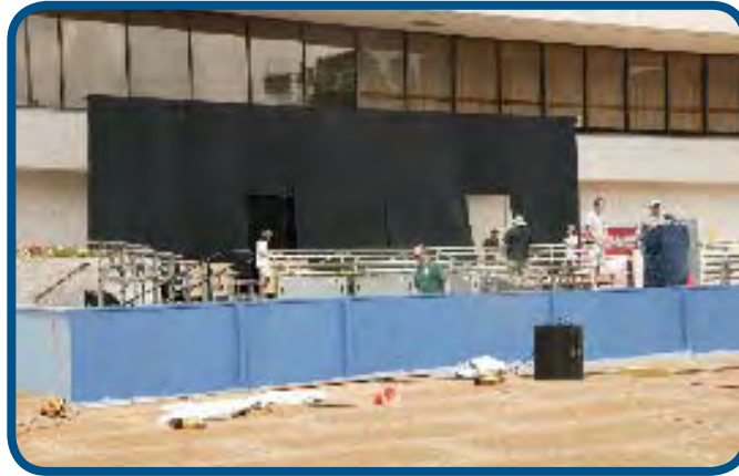
Work crews started from scratch with plywood ...
