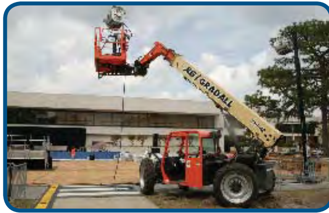
Lights were brought in as work continued overnight.
