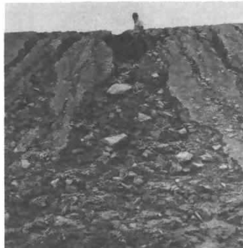
Figure 1. Ineffective reclamation. This site shown above was regraded, seeded and planted, but there was no topsoil replaced, and severe erosion has occurred on the long slopes.
