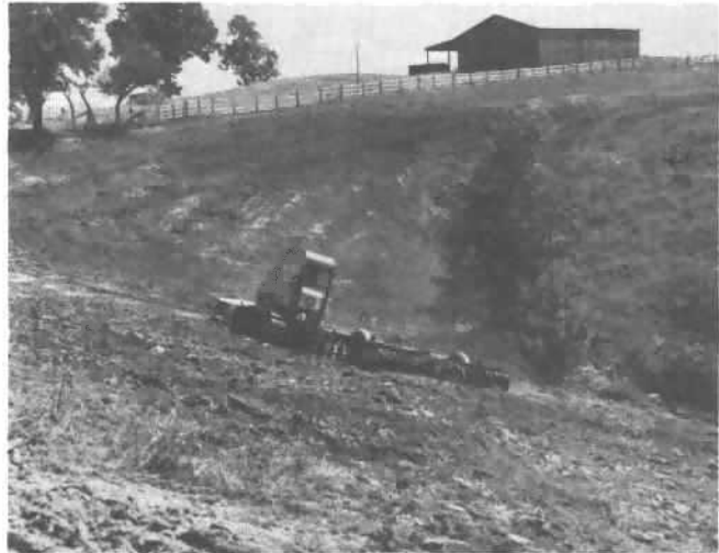
Breaking Up Excessive Compaction
