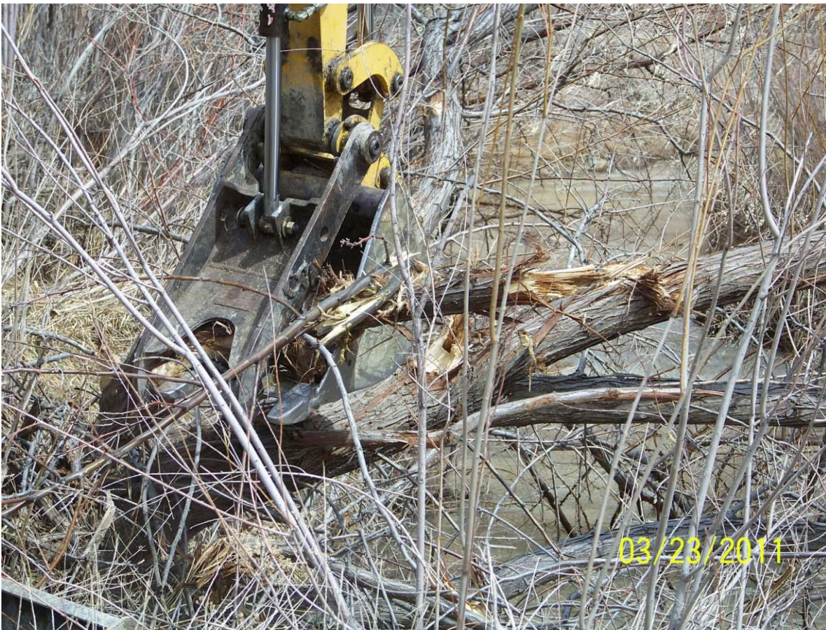
Figure 16 – Heavy equipment removing Russian olives from a Utah railroad right-of-way
