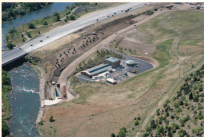
Durango Pumping Plant – Durango, CO
