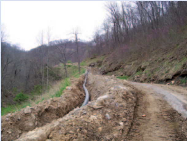
Digging the trench for the slurry line
