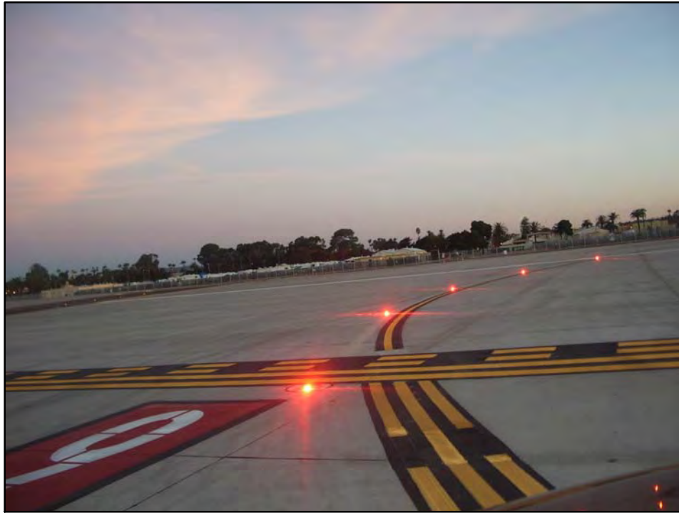
FIG 2-1-12 Runway Entrance Lights
