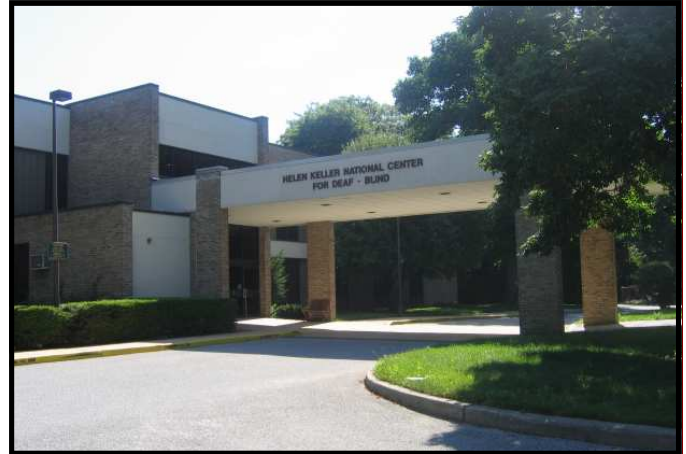
The Training Building
