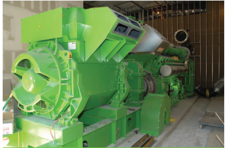
U.S. Marine Corps Logistics Base Albany will use this 1.9 MW methane power generator as part of an ongoing landfill gas project to exceed Federal renewable energy requirements. Photo by Pamela Jackson, United States Marine Corps
