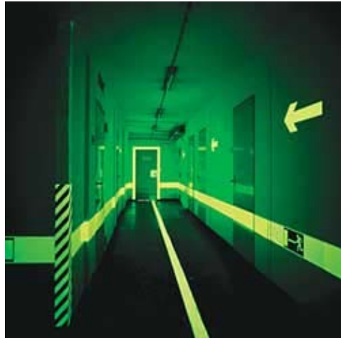
Examples of photo luminescent tape used in darkened areas denoting exit routes
