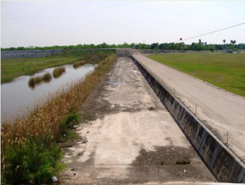
Banker Weir before diversion
