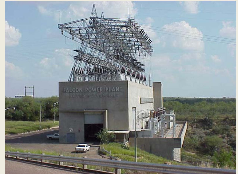
Falcon Dam Powerplant
