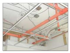
A sprinkler system designed and installed in accordance with NFPA 13R may not be used to increase the allowable area of a multifamily residential occupancy.
