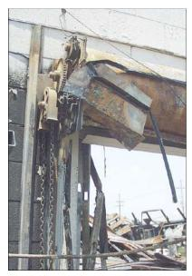
This fire door assembly failed during the Super Sofa Store June 18, 2007 fire. Photo courtesy NIST Building and Fire Research Laboratory.
