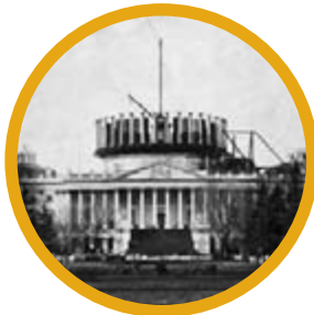
Construction of the Dome
