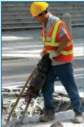
A construction worker operating a jack hammer.
