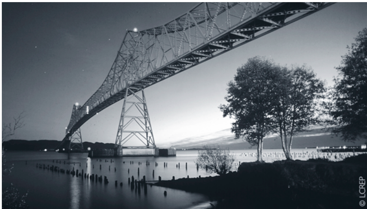
Astoria Bridge (LCREP).
