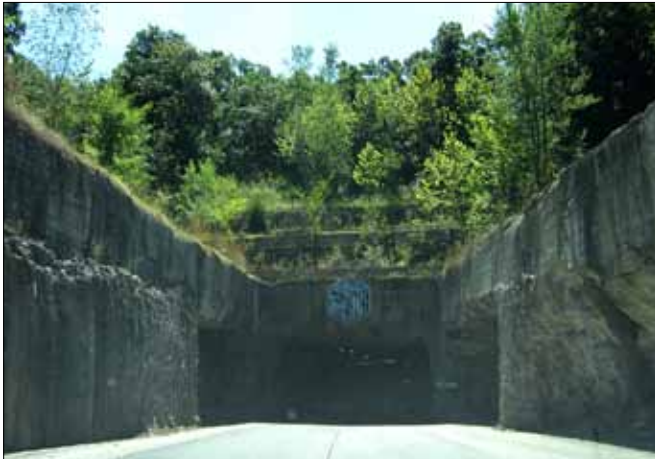
In this excavated limestone mine near Lee's Summit, Missouri, are Bennett Packaging and several other businesses, nestled next to 4 million-year-old limestone columns.
